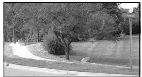
A new sidewalk was recently installed at the intersection of Beck and Powel Roads.
