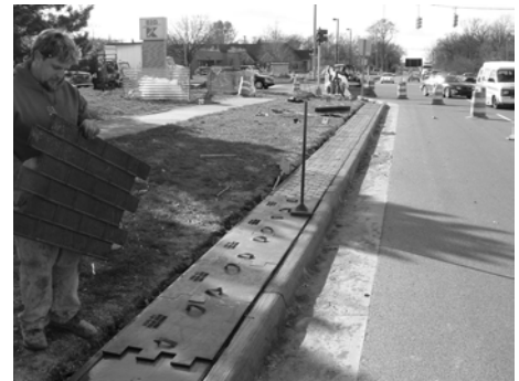
A stamped concrete verge is being installed along the Ann Arbor Road corridor (above). New sidewalks will help to make the area more pedestrian-friendly (below).
